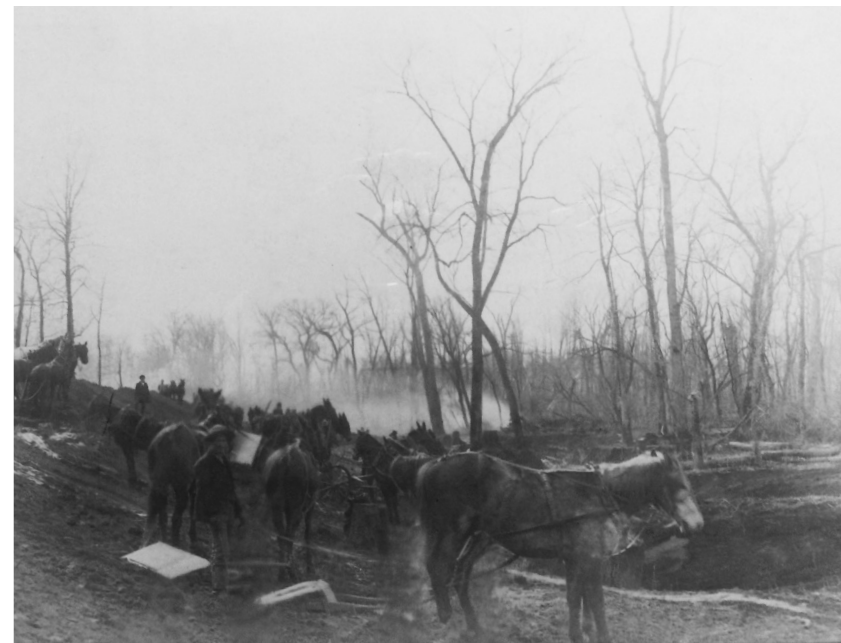
[Fig. 42] 1888 Brevoort Levee construction with slip-scrapers (in library)
